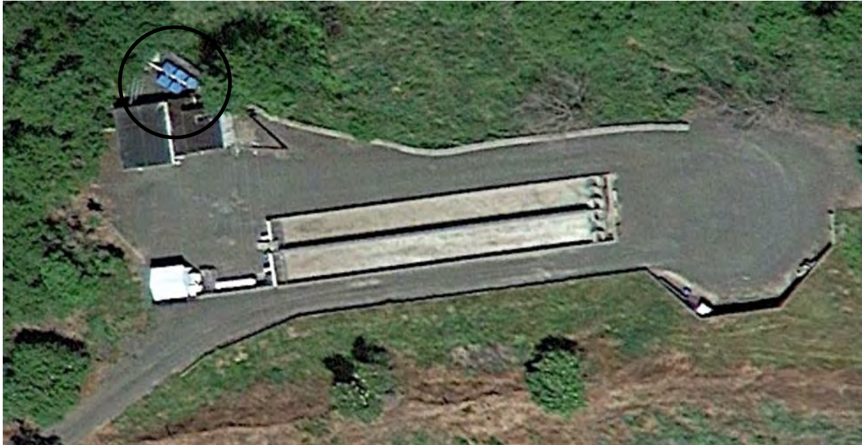
Figure 5-9. Existing Minthorn Springs Adult Lamprey Holding facility. Adults are held in tanks located in the black circle.
