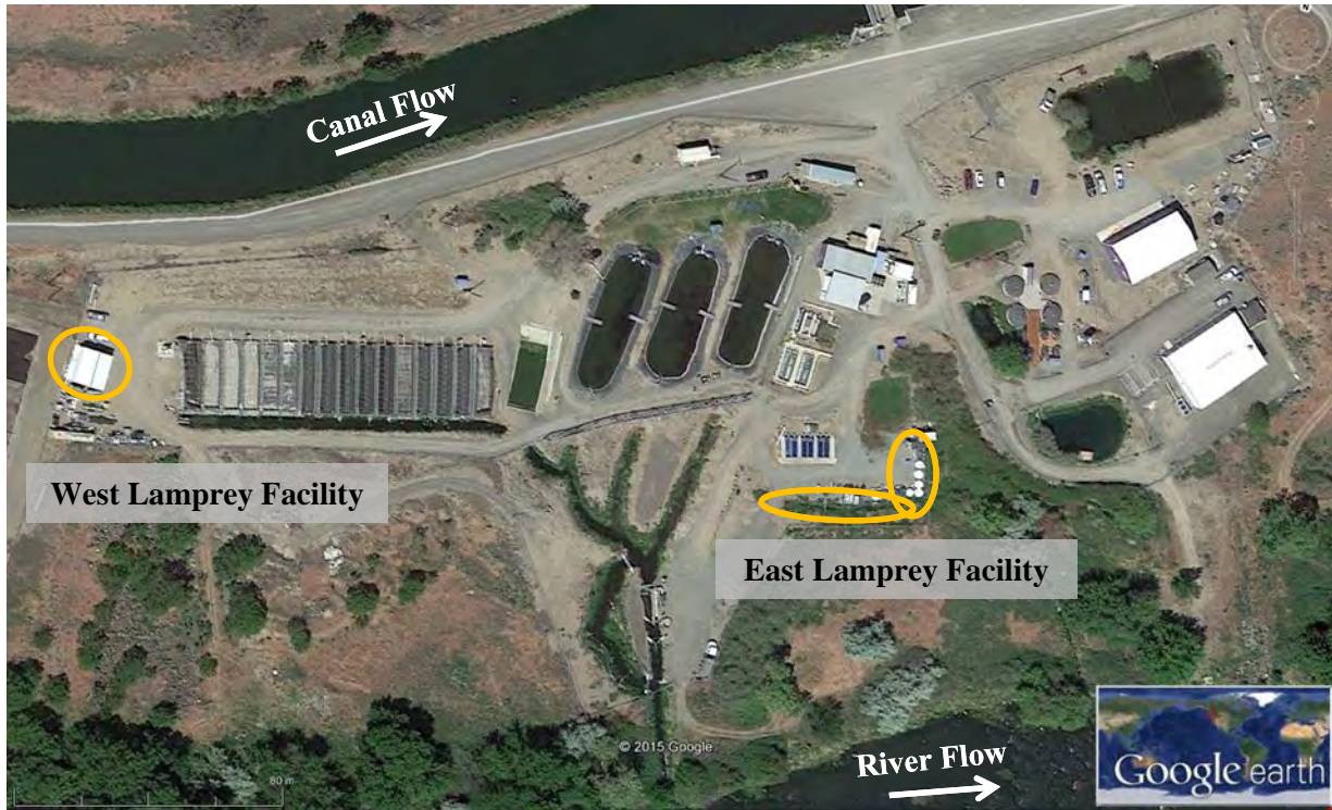
Figure 5-4. Existing Prosser Fish Hatchery aerial overview. Orange circles highlight the West and East Lamprey Facilities.
